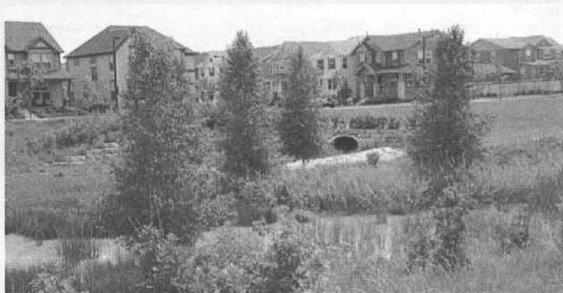
FIGURE 5-56 A consolidated treatment area adjacent to one of several neighborhoods that have been constructed as part of the project's build-out.
