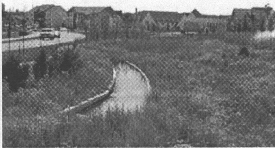
FIGURE 5-57 View of a sediment trap and porous landscape detention area in the central parkway spine of Heritage Park. The sediment trap in the center left of the photo was designed for ease of maintenance access by city crews with standard city maintenance equipment. Courtesy of SRF Consulting Group, Inc.
